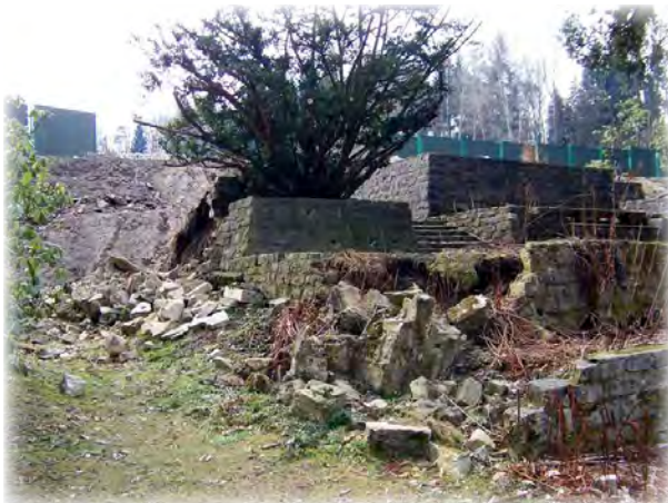
Wincenz Priessnitz heritage in the border area (before revitalisation)
