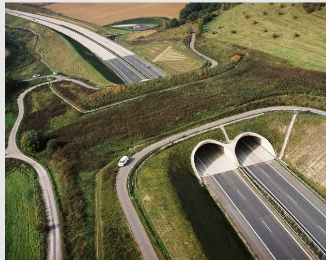
Picture No. 13: Ecological bridge "Landschaftsbrücke Meuschaer Höhe" crossing required to protect environmental use of landscape by wildlife Steel-concrete bridge, practically a tunnel, section 90 m
