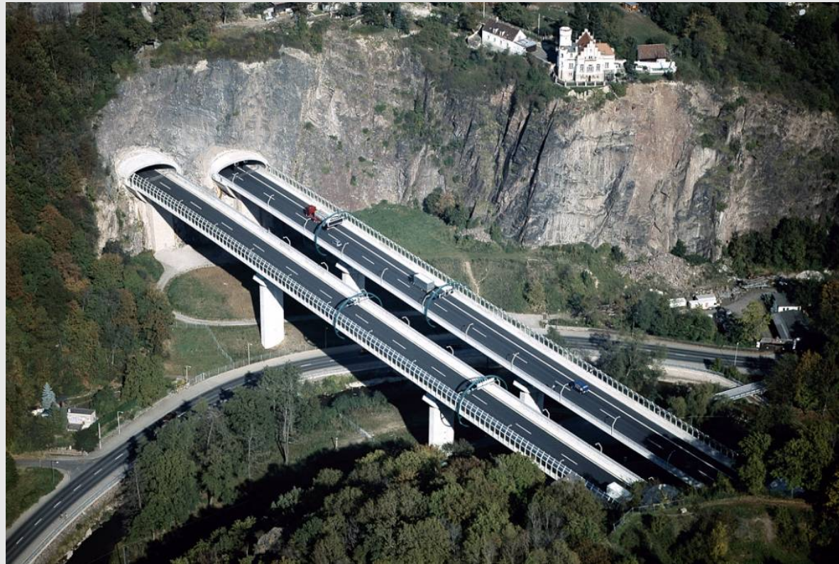
Picture No. 14: South portal of Tunnel Dölzchen and connecting Bridge over Weißeritz-Valley (A 17) Girder bridge, two superstructures, steel-concrete bridge, length 218 m, height 35 m
