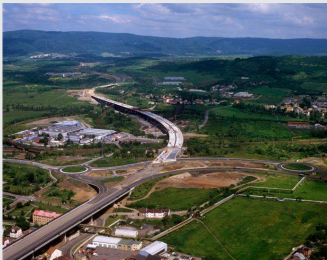
Picture No. 12: Part 0807 of D 8 starts by Trmice bridge constructed on original dumping hoppers coming from opencast collieries A typical town crossing connecting D 8 to four lanes roadway to Usti nad Labem
